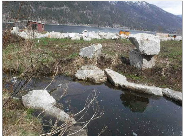
Photo 26. Newly constructed pond with rock placed along bank and instream.
