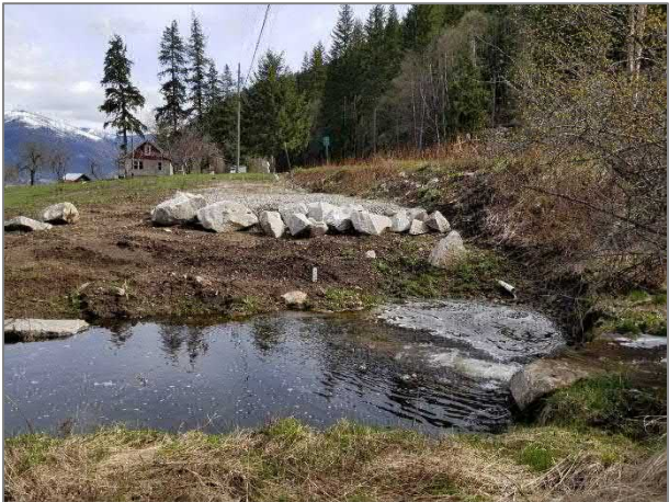
Photo 25. Newly constructed gravel parking area and constructed pond.
